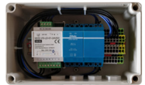
LIFT control box
