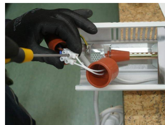
Separate the tube, unscrew wires of the emitter
